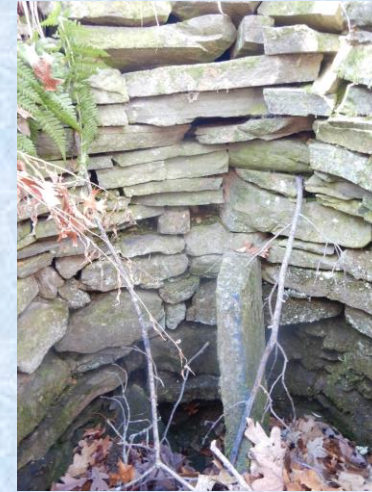
Inside dug well
