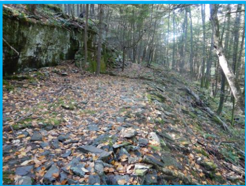
Engineered rubble roadbed.
