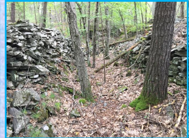
Roadway between laid rubble walls.
