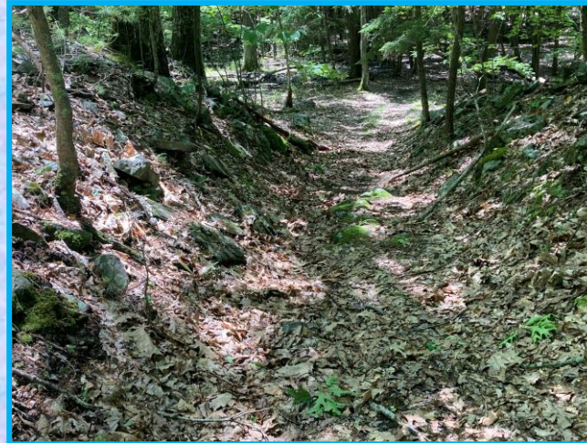
Roadway trenched through glacial knoll.
